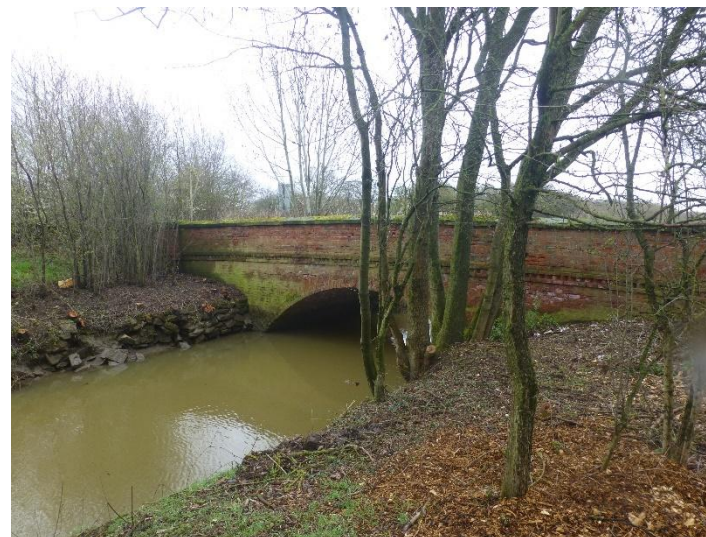
Plate 22: View of bridge adjacent to Dirtiness Cottage
