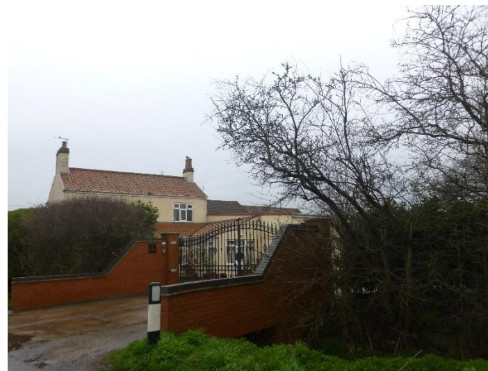
Plate 57: View of The Willows, looking north-east
