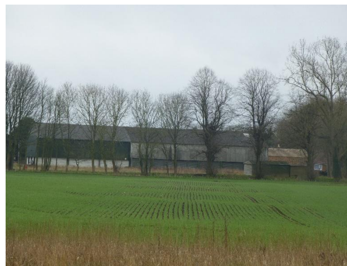
Plate 36: View of Belton Grange looking south
