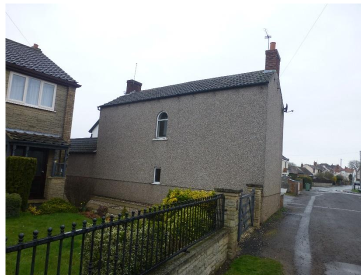
Plate 33: View of 6 Marsh Road looking east
